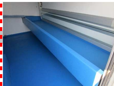
GRP pan behind the cowl, with flow holes and round corners
